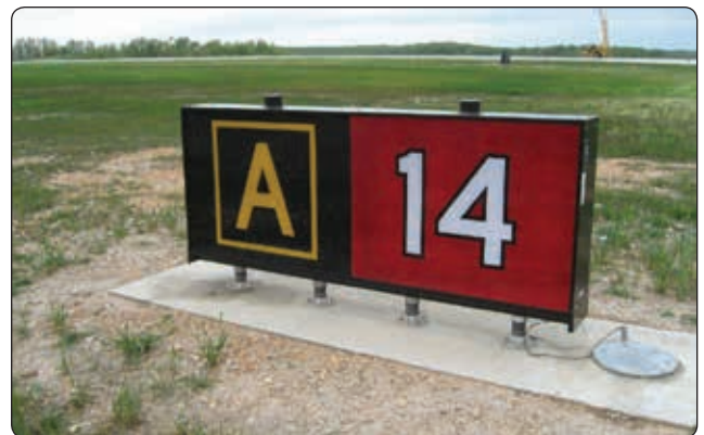
Figure 14-9. Runway holding position sign at takeoff end of Runway 14 with collocated Taxiway Alpha location sign.
