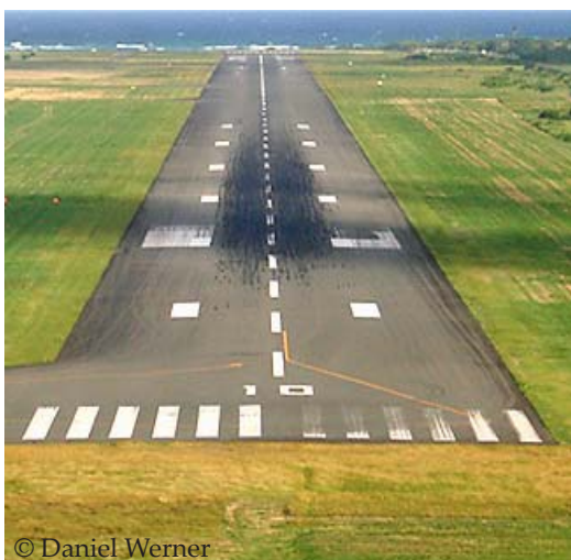
Figure 20.5a: Pattern "A", basic plain markings.
